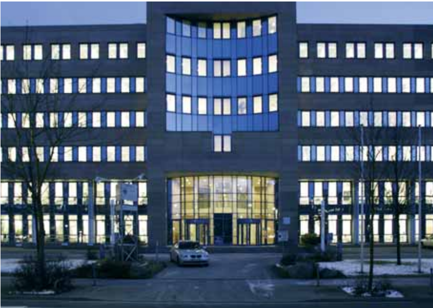
BaFin building on Lurgiallee, Frankfurt
